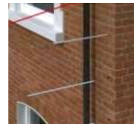
Repairing Cracks at Corners
