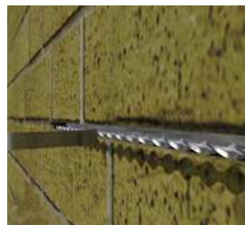
Creating Masonry Beams
